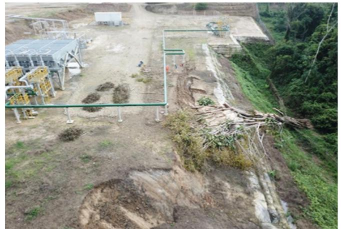
Figure 1: Slope failure area
