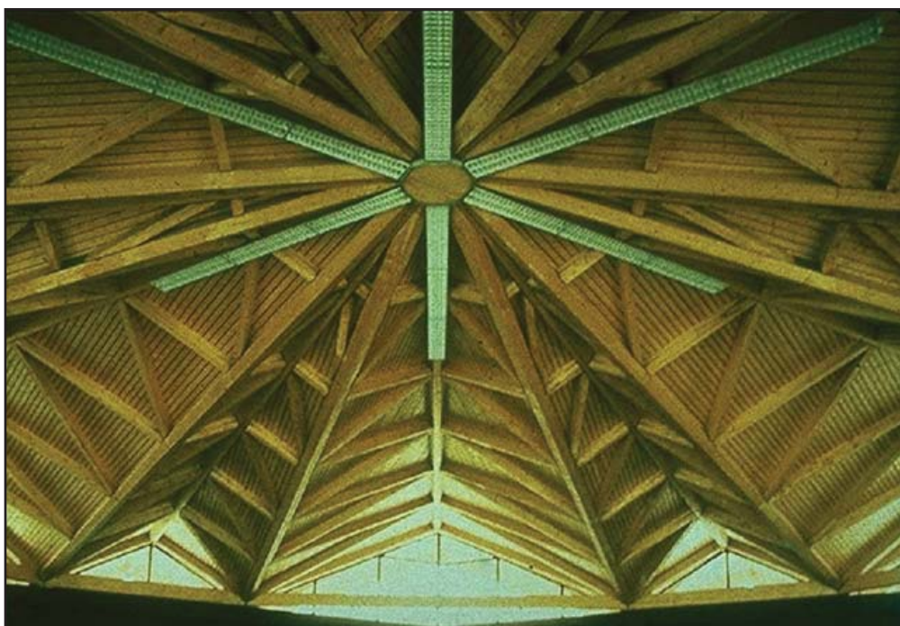
Figure 2. Folded truss structure Hartwald Clinic Pavilion, Bad Zwosten Germany, architect A. Frank, the designer of the construction Natterer, 1977.
