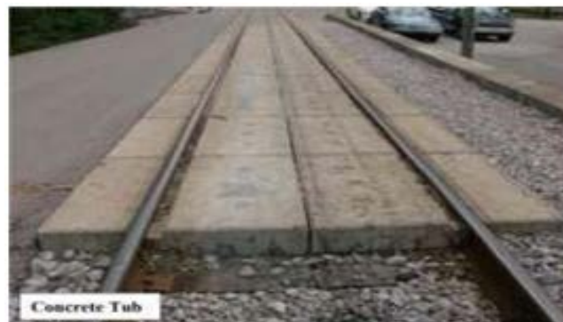
Fig. 8. Type of Concrete Tub [3]
