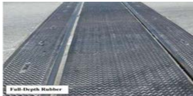
Fig. 7. Type of Combination Surface [3]
