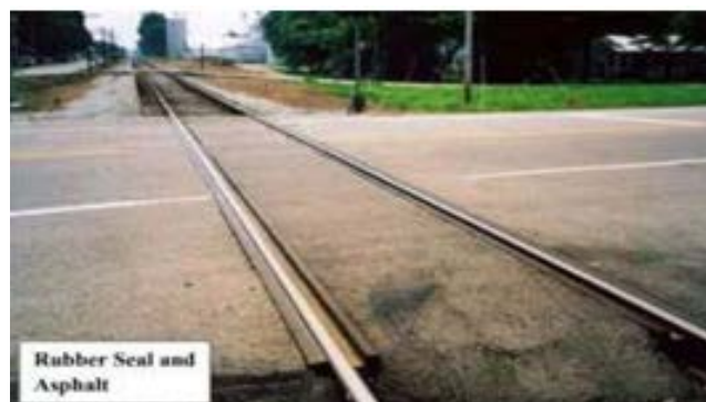
Fig. 3. Type of Rubber Seal and Asphalt Surface [3]
