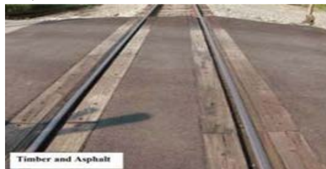
Fig. 2. Type of Asphalt Surfaces on Rails [3]
