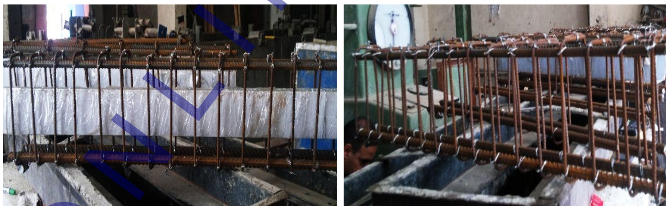
Fig. 2. Reinforcing bars and plastic pipe
