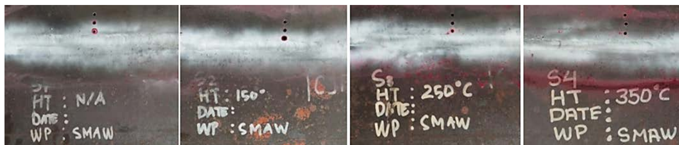
Fig. 7. Visual and liquid-penetrant inspection results of SMAW-welded joints under no-preheating, 150 °C, 250 °C, and 350 °C conditions
